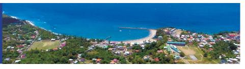
At the time of this writing, heavy seas were causing waves to break at the end of the unfinished breakwater, although the completed structure should remedy this. There were not yet any channel markers, and although the lagoon was recently dredged to 15 feet, shoaling is still occurring at an unknown rate —
